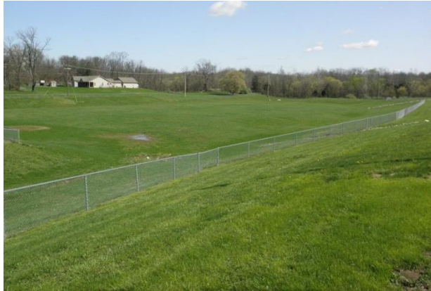
Storm Water Retention Pond
