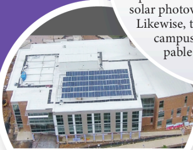
Rockville Campus Science West Photovoltaic Array
