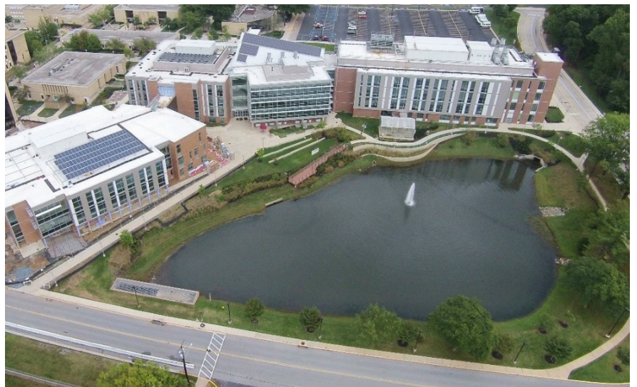
Science Center (SC) on the Rockville Campus (top right) LEED Gold Certified, Science East (SE) (middle) LEED Gold Certified, and Science Center West (SW) LEED Gold Targeted (bottom left)
